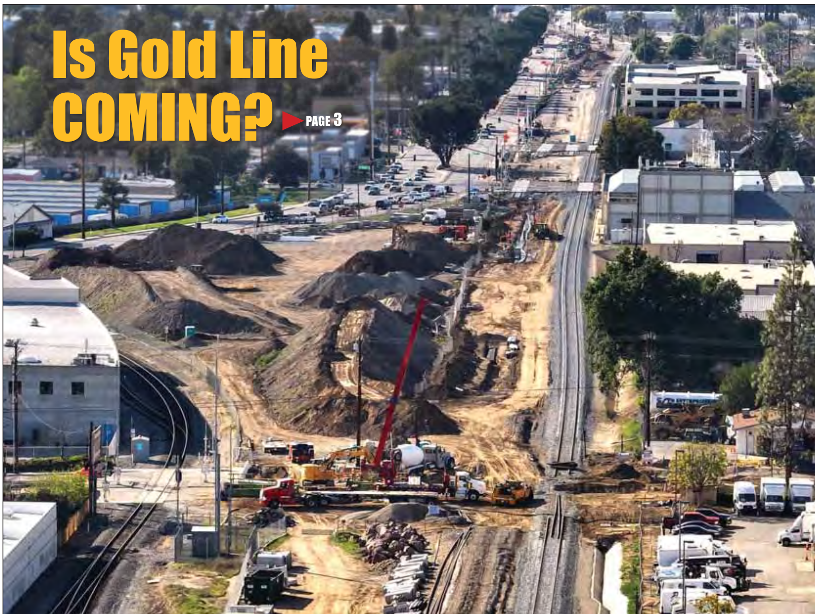
On Wednesday, a work crew constructs the future Gold Line light rail tracks near the intersection of White Avenue and Arrow Highway in La Verne. Under current funding the Gold Line's terminus will be at Pomona North, however, Claremont Mayor Pro Tem Ed Reece recently sent a letter to Sacramento requesting funding to bring it through Claremont and Montclair. COURIER photo/Peter Weinberger
