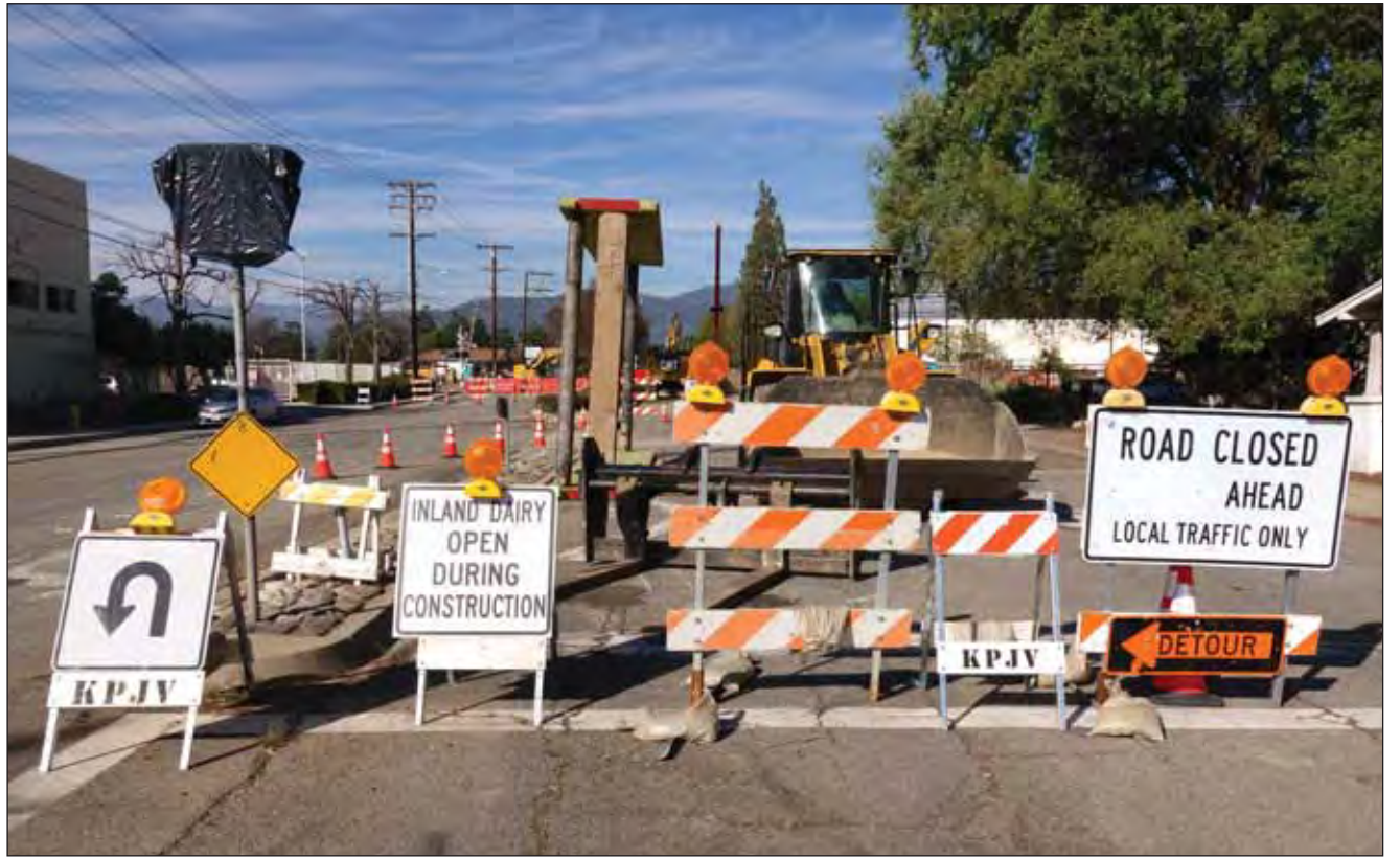
White Avenue in La Verne is blocked to all traffic to accommodate Gold Line construction headed east towards Garey Avenue. COURIER photo/Peter Weinberger
