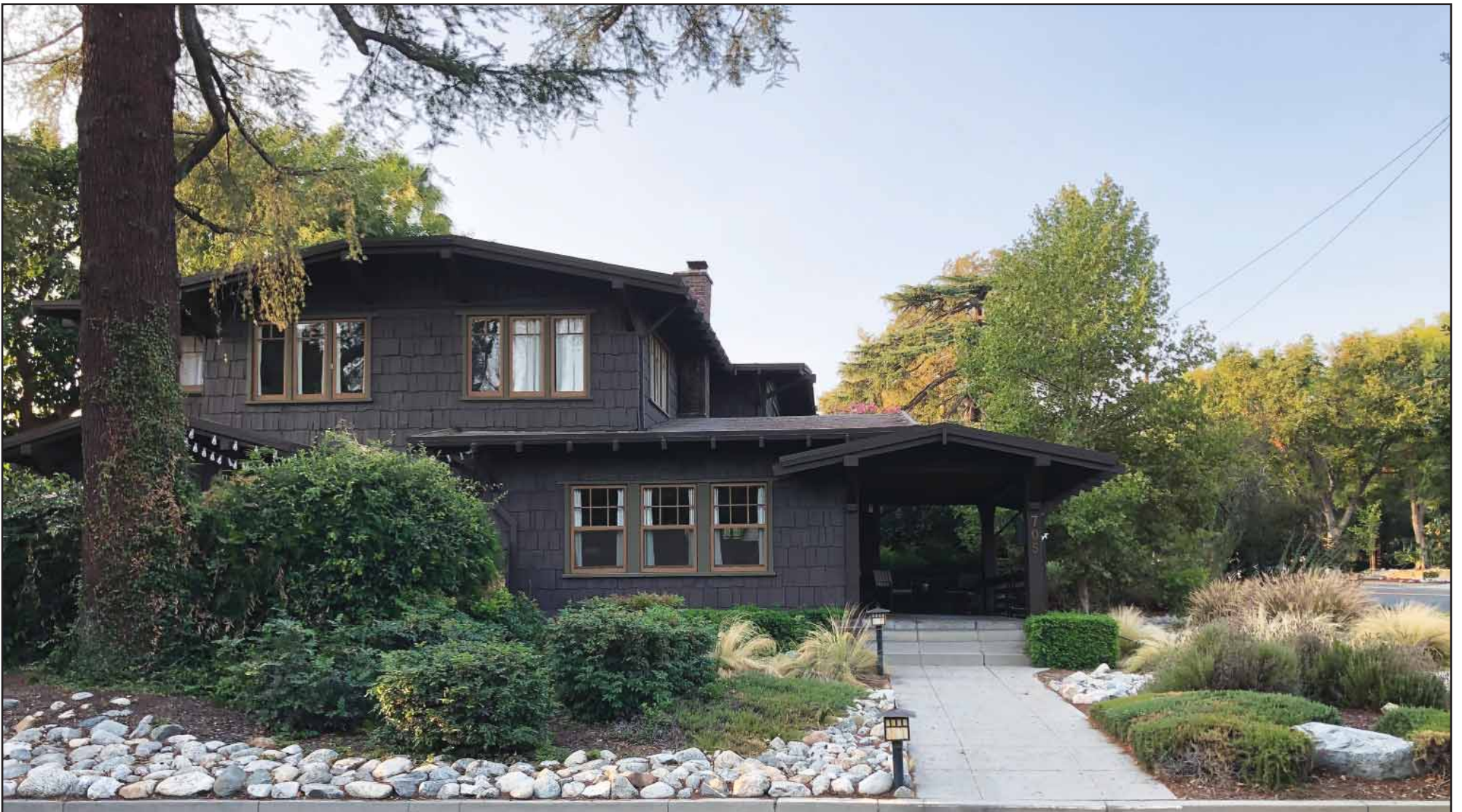
This home on Indian Hill Boulevard features low-pitched, gabled roofs common to the California Craftsman style. Photos/courtesy of John Neuber
