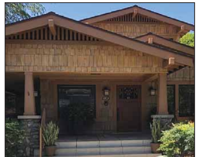
The one-story porch of this Craftsman home on College Avenue projects from the house with a gabled roof and is indicative of the style.
